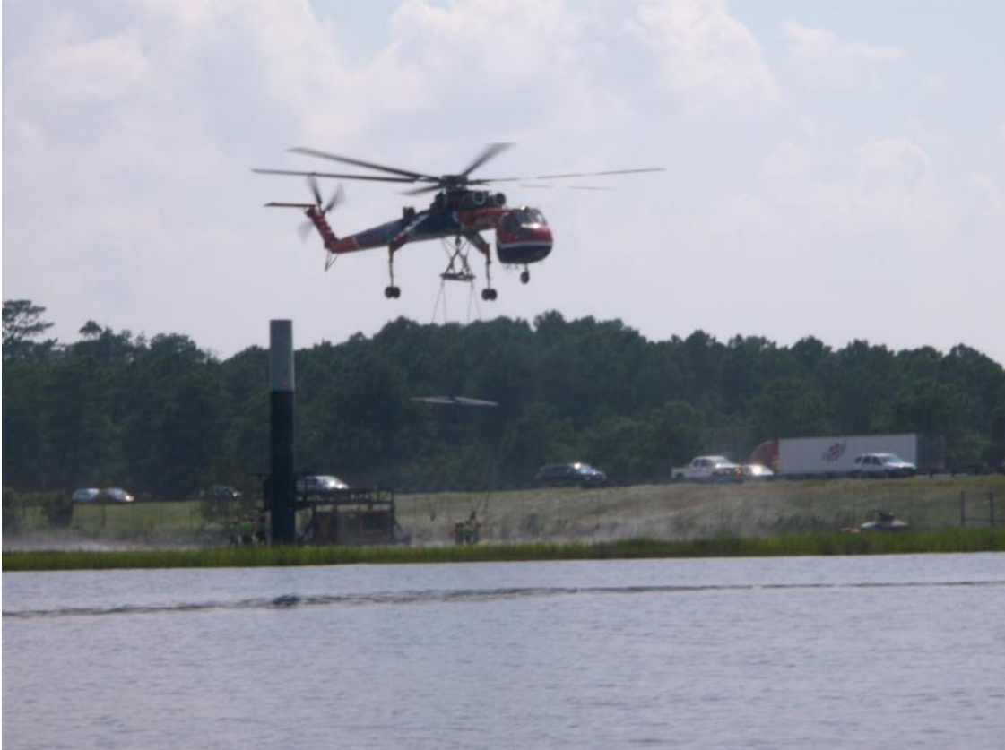
Helicopter installing power poles across waterway
